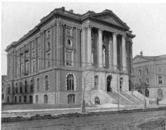
ROGERS BUILDING Massachusetts Institute of Technology
